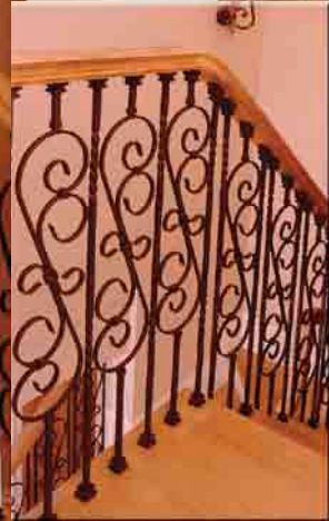
A very subtle transition from the rake handrail to the level handrail at the second floor is achieved with our overreasing handrail fitting.
