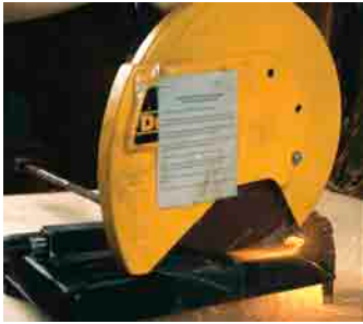
Step 1: Mark and trim each baluster from the bottom.
