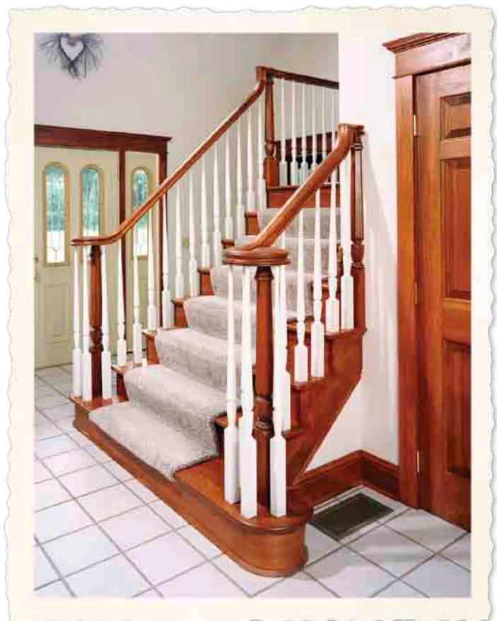
Pictured: LJ-6400 Handrail, LJP-30108 Utility Newels, LJP-30148 Utility Newel, LJP-30148 Utility Newel (half), LJP-20158 Balusters, LJ-7430 Left Hand Volute, LJ-7435 Right Hand Volute and 2 Landing Fitting Assemblies.
