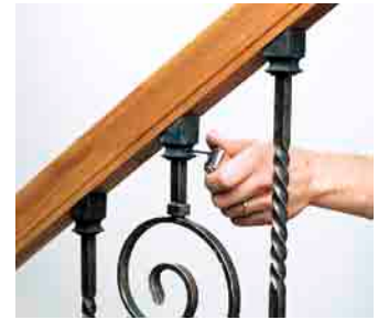
Step 7: Using an allen wrench secure each top base against the rail and each bottom base against the tread.
