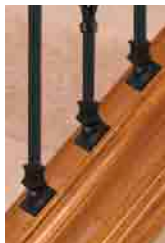
Kneewall Stair Bottom Connection
