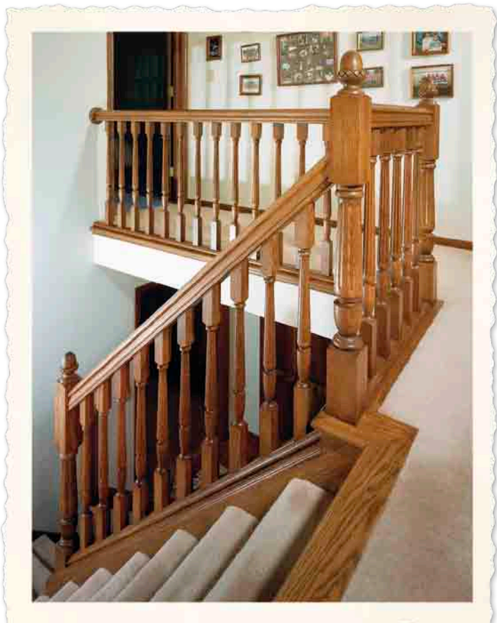
Pictured: LJ-6519P Handrail, LJ-6006 Shoerail, LJ-6007 Fillet, LJF-3046 Intermediate Landing Newel, LJF-3045 Second Floor Landing Newels, LJF-2005 Balusters and LJ-7026 Rosette.
