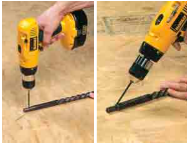
Step 2: For rake balusters, drill a hole perpendicular through the top pin on every 6th baluster. For balcony balusters, drill the hole at an angle.
