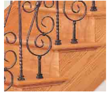
Step 4: Apply construction adhesive in the predrilled holes in each tread. With a bottom base on each baluster, place all balusters in position on the treads. *Below left are alternate methods for securing iron balusters to the treads.
