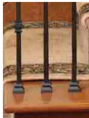
Open Tread Bottom Connection
