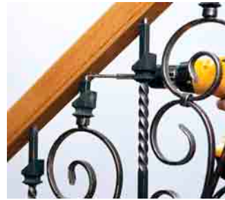
Step 6: Securely attach every 6th baluster to the handrail using a flat self-tapping screw. Smooth the screw head with emery paper, then spot putty for painting.
