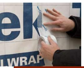
Taping the seams after wrapping is the best practice for completely sealing the building envelope.
